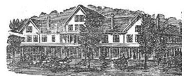
The Crawford House, Crawford Notch, the White Mountains, New Hampshire.
